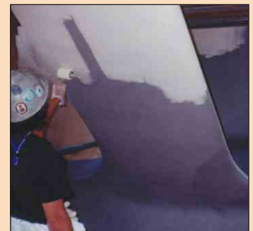
Large scale application to virtually any rigid surface prior to painting.
